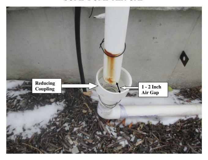
This is a photo of an air gap installation on a sump pump discharge line. This prevents backpressure on the pump in the event the exterior line freezes or becomes clogged on the exterior drainage extension.
