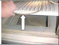
It can be difficult to remove and insert the filters due to access and filter brackets.
