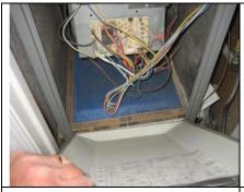
With an up-flow furnace, the filter can be located in the blower motor cabinet.
