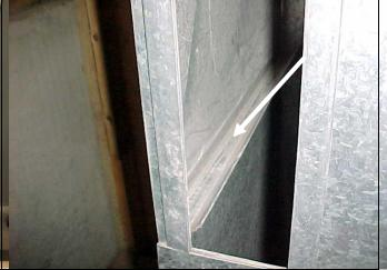
There is a ledge that the filter sits on for the diagonal filters, it is important to set the filter properly on this ledge.
