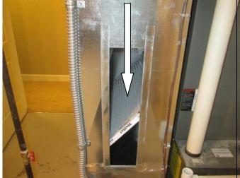
Some filters are installed diagonally and the airflow is down the return ductwork in the vertical direction.
