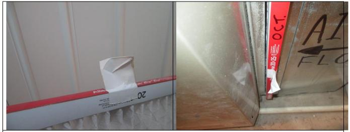
Some filters fit into the duct work without providing an edge to grasp for removal. I recommend using a piece of duct tape on the end which will provide a tab to grasp for easier removal.
