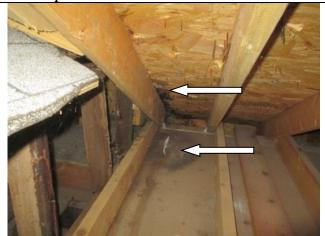
Water damage and mold/mildew growth on the interior drywall and wood framing and roof decking can be clearly seen here.
