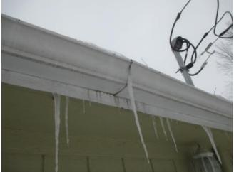
Ice dams formed in the gutters and backed up on the perimeter of the roof.
