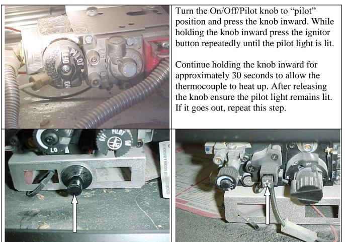
Two types of ignitor buttons are shown here. You can test the ignitor buttons prior to turning on the pilot. You should see a blue spark in the fireplace (near the pilot gas supply orifice) each time the button is pressed. If you cannot see the spark, try turning off the lights in the room.
