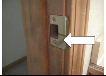
If the latch is missing low on the strikeplate insert the 3 inch screw in the lower hinge center hole.
