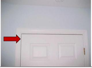
If the door sticks at the 'top-side' insert the 3 in screw in the upper hinge center hole.
