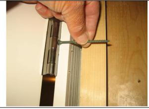
A 3 inch deck screw will go through the door jamb, rough opening and into the 2x4 framing where it will pull the hinge inward and adjust the door.
