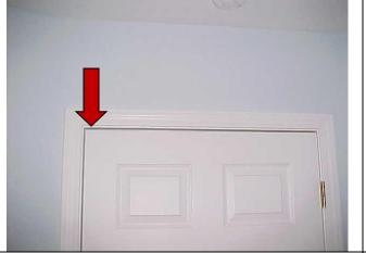
If the door sticks at the "top-top" insert the 3 in screw in the lower hinge center hole.
