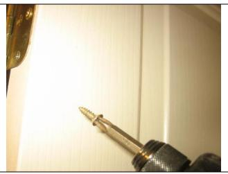
This <sup>3</sup>/<sub>4</sub> inch screw barely penetrates through the jamb and does not secure the door to the framing. Over time a door may move out of plumb for any number of reasons (sag, shrink/swell of lumber, etc.)
