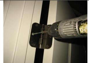
Install the 3 inch screw in the center hinge hole. This lines up the screw towards the center of the 2x4 and minimizes the potential that the 2x4 splits on the edge.
