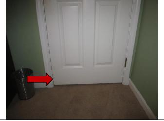
If the door sticks at the 'low-side' insert the 3 in screw in the lower hinge center hole.
