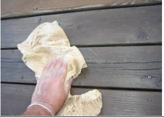
After application with a brush, rub the sealant in with rag to get better penetration and minimize wet spots.
