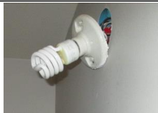
Missing/broken cover plates on switches, outlets, junction boxes and fixtures need to be installed and secure.
