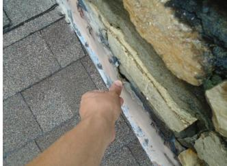
Close up of step flashing caulk that has deteriorated causing water penetration into the attic. This caused saturated insulation and interior wall and ceiling damage.
