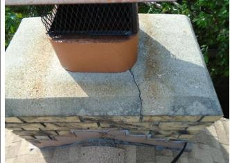
Some cracks are large enough that you can apply a polyurethane caulking to fill cracks prior to applying the brush on sealant.
