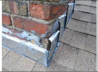
This photo shows a chimney with the proper flashing installed poorly. Note the counter flashing is not secure against the brick and the top is not sealed in the masonry joint.
