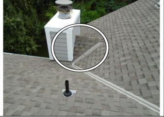
A chimney cricket is a 'peak' at the center of the chimney base that diverts water and minimizes the potential for snow accumulation. A cricket, as shown here, is recommended for any span over 30 inches.
