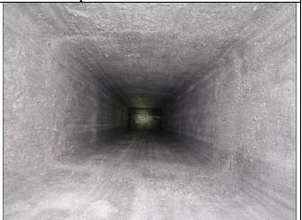
Photo of a relined chimney completed instead of installing a steel liner. This type of repair is completed using a sprayer.
