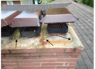
Cracks in chimney caps should be sealed brush on elastomeric sealant for long term protection. This covers the entire chimney cap and provides a waterproof seal.
