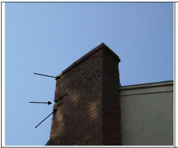
Spalling occurs when brick deteriorate and layers 'flake off' causing damage.
