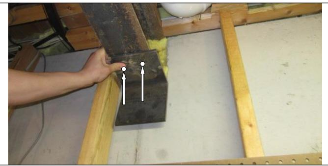
Two holes should be drilled through the angle iron and the horizontal face (flange) of the I-Beam in the position shown above. There should be on bolt on each side of the vertical section (web) of the I-Beam secured with a locking washer and nut.
