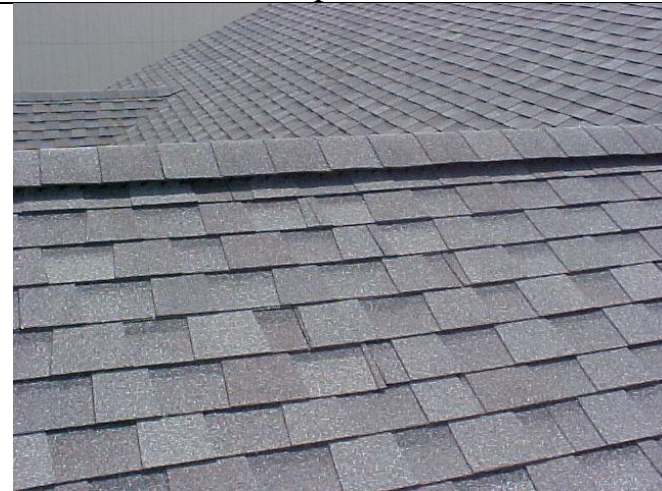
Ridge vents are becoming more popular and are designed to operate similar to roof louvers while providing continuous ventilation along the length of a roof.
