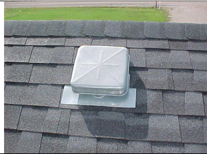
Roof louvers are low profile vents installed near the peak of the roof that allow hot air to escape.
